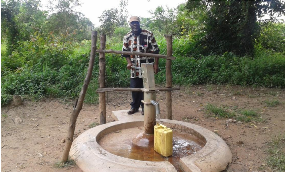
MFS II evaluator on the newly constructed borehole in Gwengdiya parish, Awach Sub County
