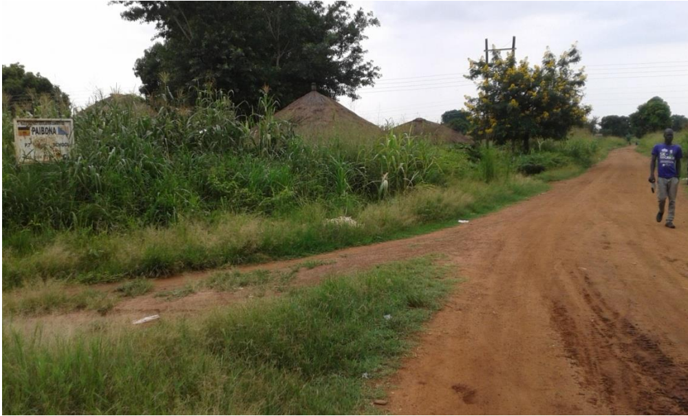
The rehabilitated Awach – Paibona road which is about 12km
